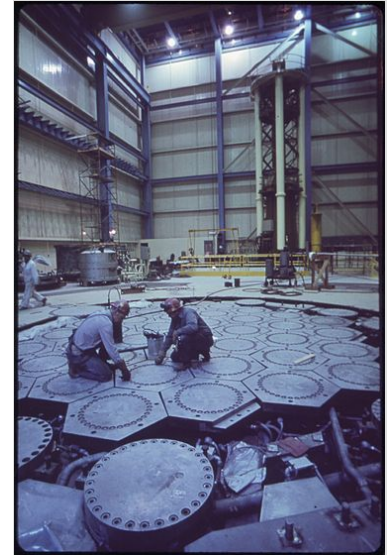
Refueling floor at Fort Saint Vrain HTGR, 1972
